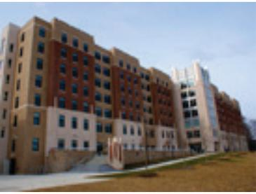
Thin brick, precast sandwich panels provide “collegiate Gothic” style to Catholic University of America’s Opus Hall.
