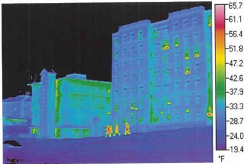
Illustration 6. In contrast to illustration #5, this thermal image of the precast concrete wall system at Opus Residence Hall at Catholic University of America indicates that little heat is escaping anywhere in the building's wall system. Photo: Little Diversified Architectural Consulting
