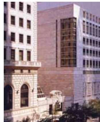
Stone veneer-faced precast panels clad the Federal Reserve Bank in Cleveland, Ohio.
