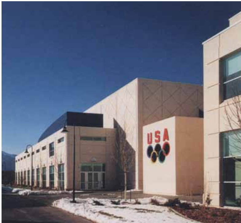
Diagonal reveals were used on the athletic portion of the Gymnasium and Aquatic Center at the U.S. Olympic Training Center, while vertical and horizontal reveals were combined on the building's two-story support section. (Courtesy ©Steinkamp/Ballog Chicago)
