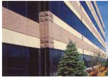
Figure 5 Multiple mixes with acid-etched and form-liner finishes.
