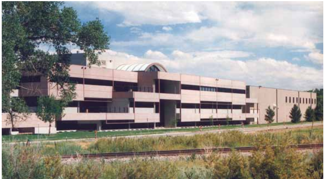
The award-winning expansion of Pfizer's Valleylab campus features flat sandblasted panels over an exposed steel structure.
