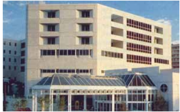
The Children's Medical Center in Dallas used precast concrete extensively in the exterior envelope. Large recessed window openings add sculptural interest to the overall mass of the project, providing significant solar shading for those specific windows.
