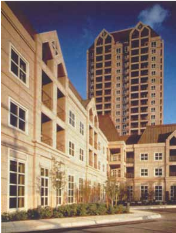
The USAA Retirement Center in San Antonio features precast concrete throughout the façade. Window panels on the low-rise structures highlight a variety of profiles and treatments, as do the balconies and window areas of the tower of the project.
