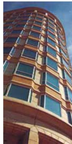
**Figure 12** This flat wall plane on the 55 Farmington building in Hartford, Conn., changes direction without corner articulation by using a shallow angle return for single casting and placing the joints at the back angles where they are de-emphasized. The shallow corner angle allows a solid cast edge.
