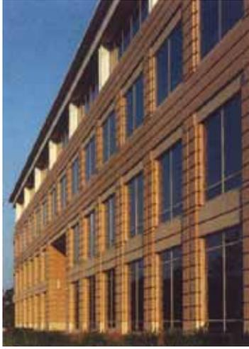
**Figure 9** The heavily rusticated panels used on 1335 Windward Concourse in Atlanta are thickened flat panels with exaggerated 3-inch quirks at the corners to create a return back into the interior of the building, giving it a perceived dimension.
