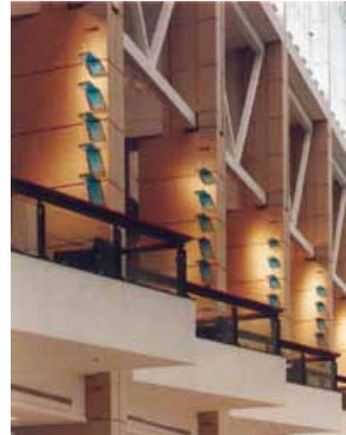
**Figure 13** The returns on these column enclosures at the McCormick Place Expansion project in Chicago aren't intended to imply a material thickness of panels or blocks but to provide a planar wrap of the surfaces forming the corner. The joint is located at the pier's center to provide a linear continuation of the element above the pier.
