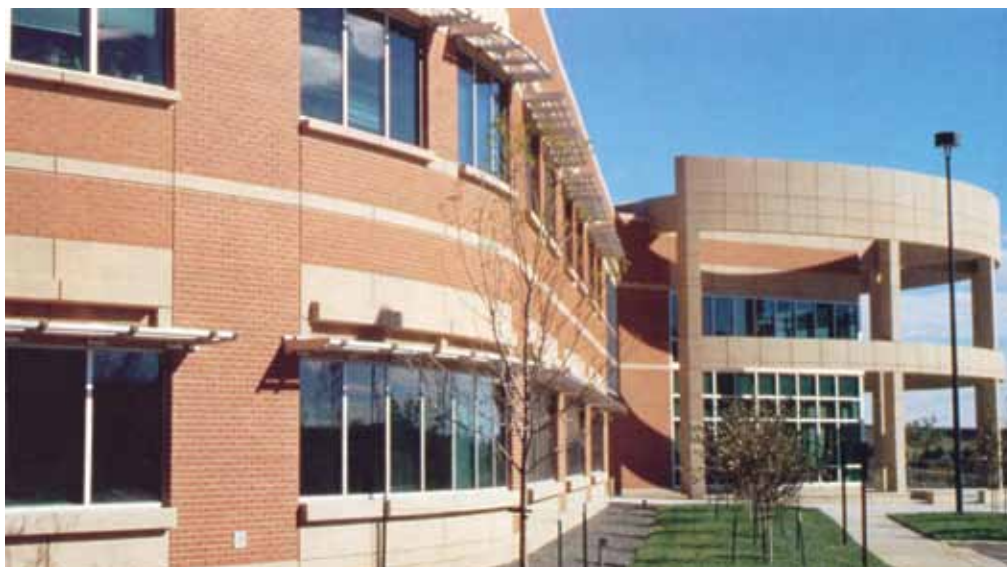
At the Jefferson County District Attorney's Office Building at Golden, Colo., the use of curved precast panels allowed the designers to repeat the radiused building corner with a curved open pergola at the entry. (Courtesy Jun Xia, Gensler)
