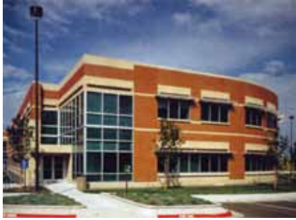
At the Jefferson County District Attorney's Office Building, masonry units cast into the precast panels provided a combination of brick and precast detailing. (Courtesy Jun Xia, Gensler)
