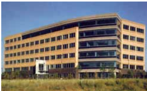
The use of curved precast panels allowed the designers to "break out of the box" at the 370 Interlocken Boulevard project in Broomfield, Colorado. (Courtesy Ed Lacasse)
