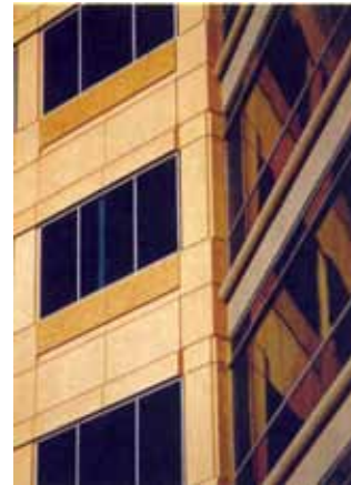
The combination of different colors and textures of precast structural spandrel panels, including radius panels, creates a highly articulated but very cost-effective façade at the 370 Interlocken Blvd. project.)
