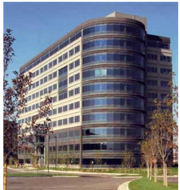
The combination of radiused structural precast panels and storefront glazing allowed designers to express a curved "glass" volume without the additional cost of the curtain wall at the 380 Interlocken Crescent project in Broomfield, Colo.
