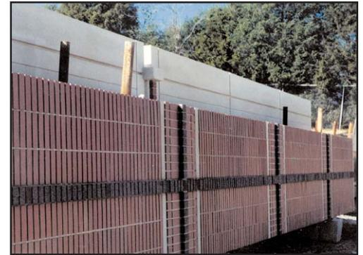
Once the panel has cured overnight, it is stripped from the mold and acid washed to remove the retarder and complete the accent strips.
