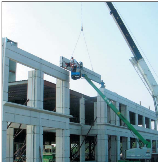
Architectural precast panels were erected in nine weeks at Deerwood North 300.
