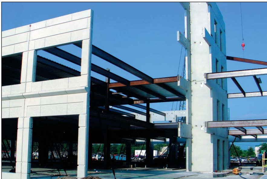
Architectural precast panels were erected in nine weeks at Deerwood North 300.
