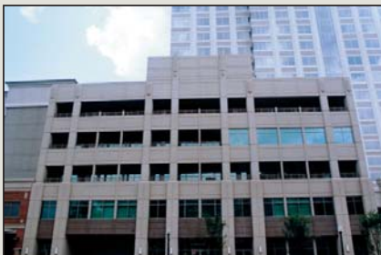
West elevation: Five-story office building
